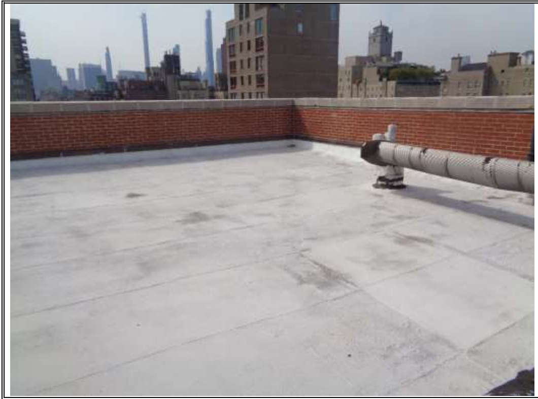
Photo 7 – View of the roof at 45 East 82 nd Street.
