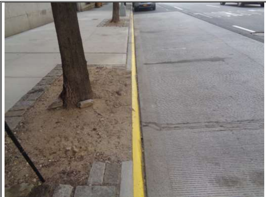
Photo 4 – View of a typical curbing.
