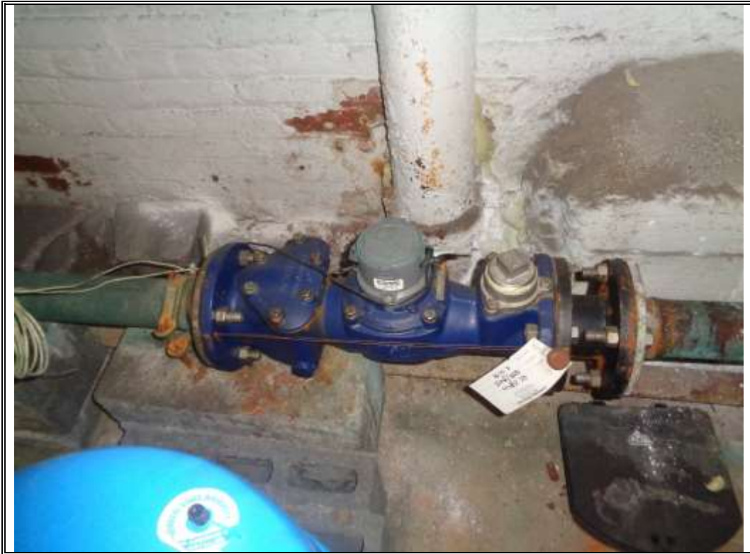
Photo 15 – View of the water meter located in 45 East 82 nd Street.
