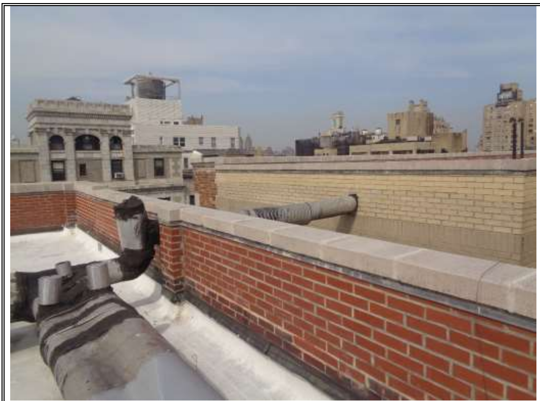
Photo 8 – View of the parapet wall at 45 East 82 nd Street.
