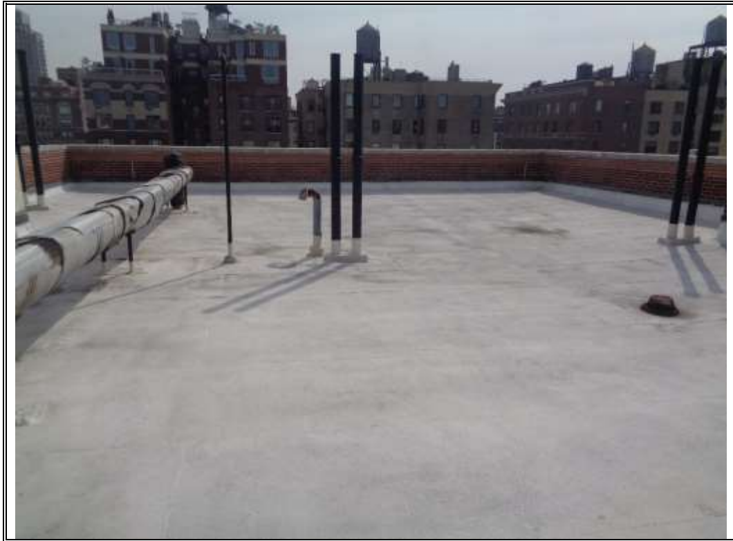
Photo 5 – View of the roof at 40 East 83 rd Street.
