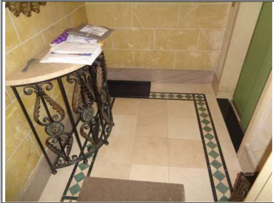
Photo 21 – View of a tenant-maintained elevator lobby.
