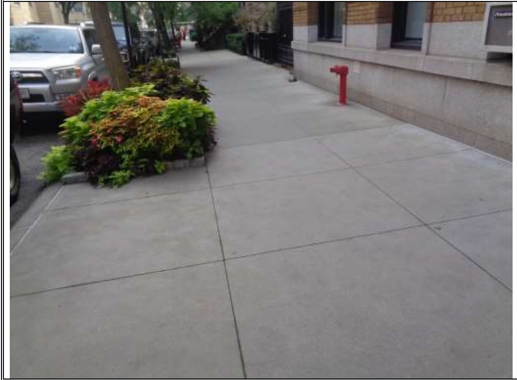
Photo 3 – View of typical flatwork condition.
