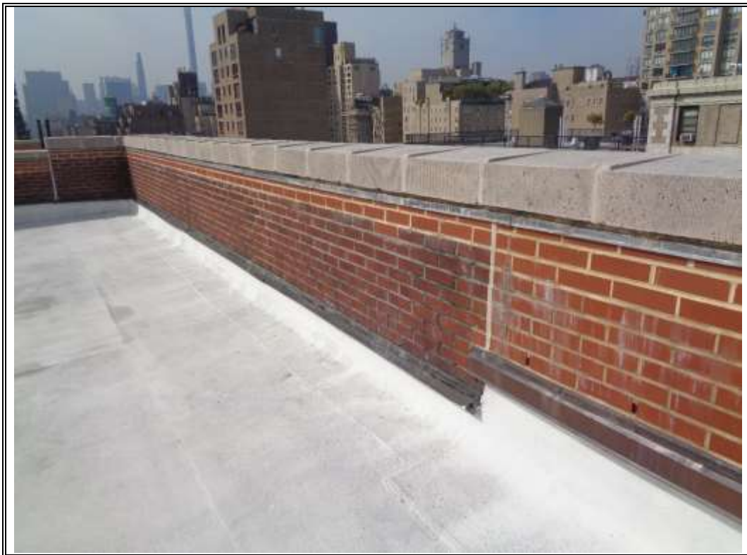
Photo 6 – View of recently repaired/ built parapet wall at 40 East 83 rd Street.
