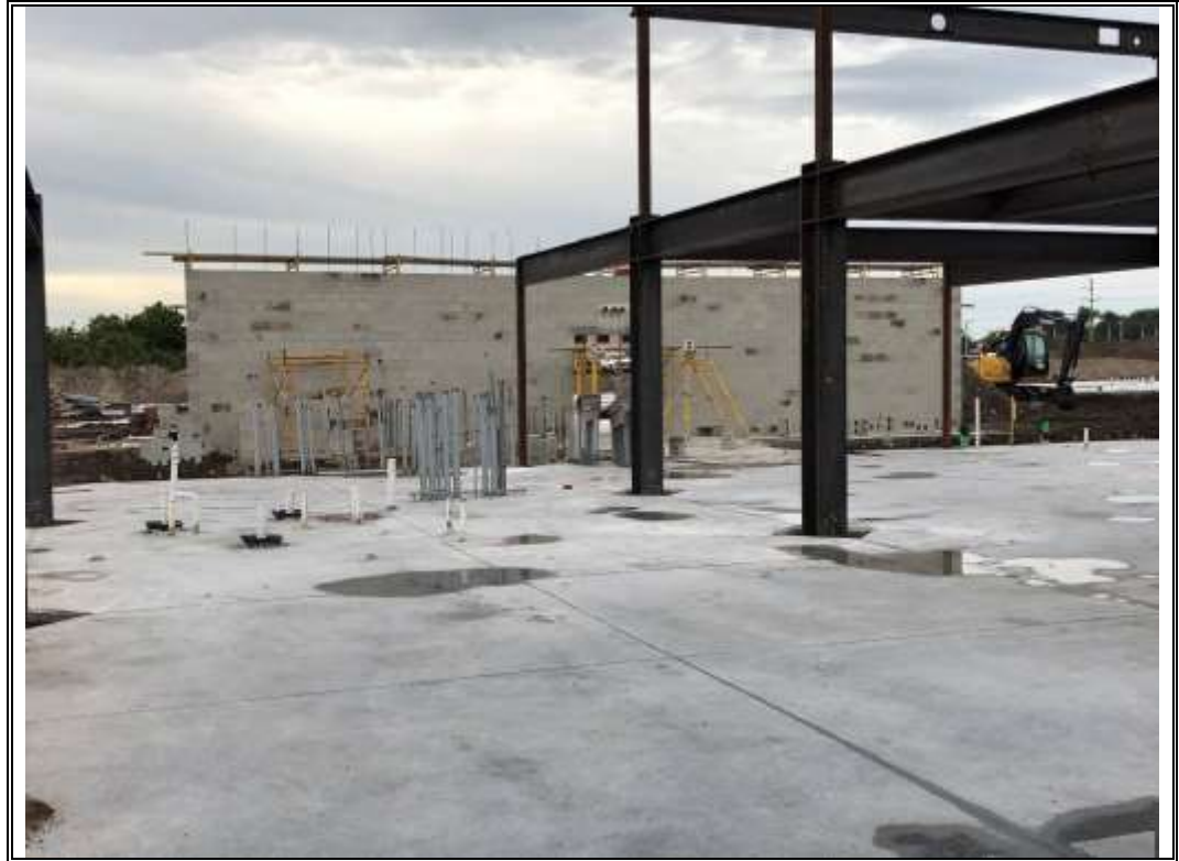
Photo 5 – View of structural steel and completed CMU.
