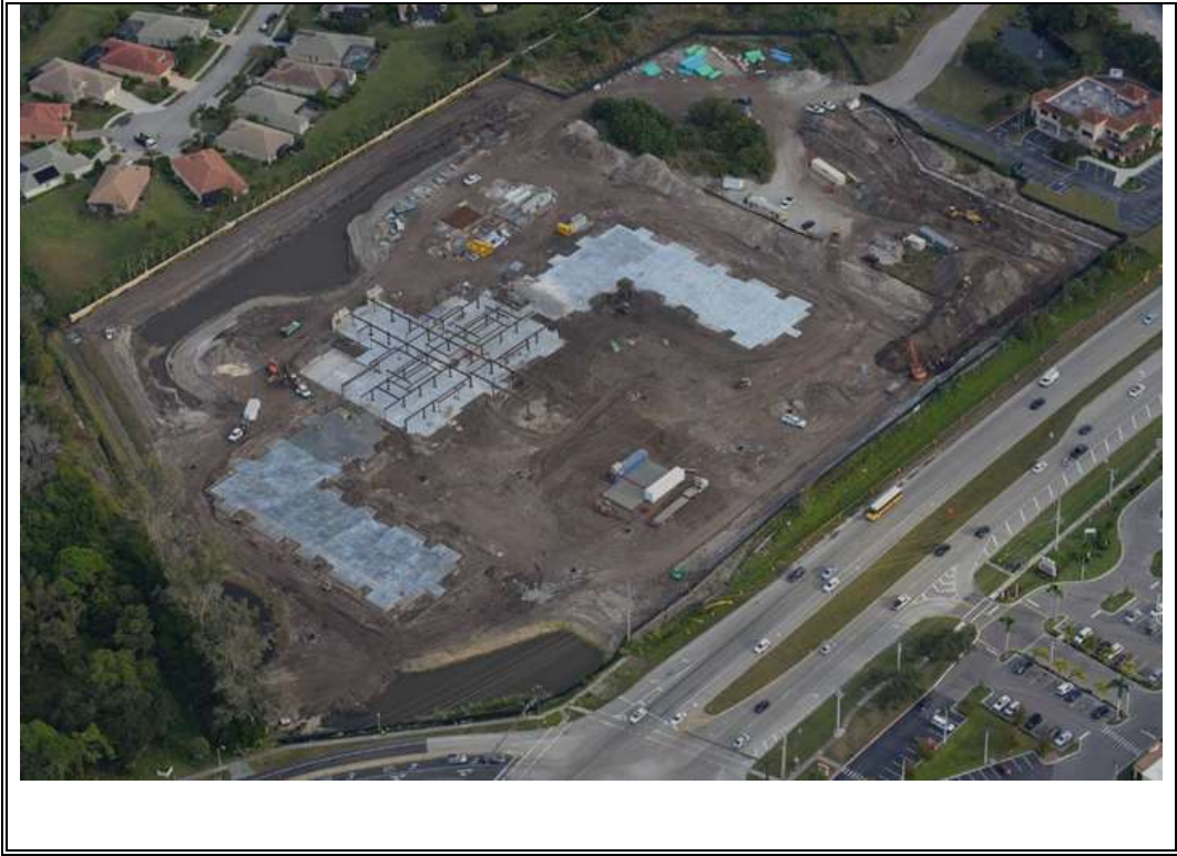
Photo 1 – Aerial view of the project. (Photograph provided by GC)
