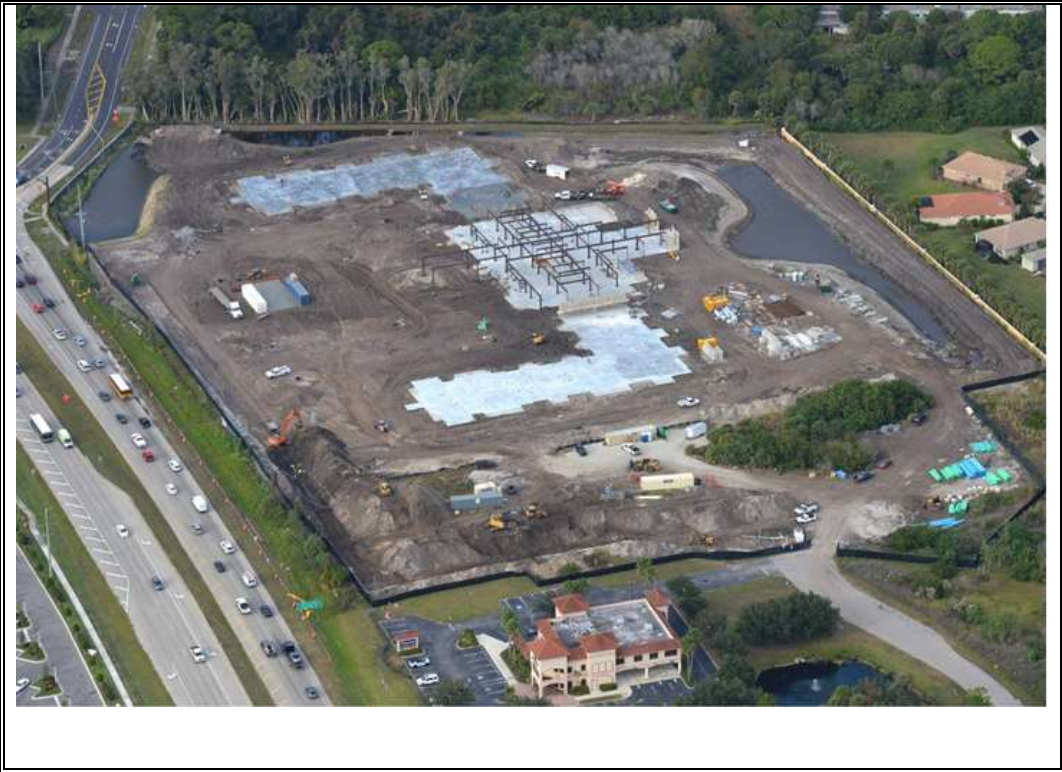
Photo 2 – Aerial view of the project. (Photograph provided by GC)
