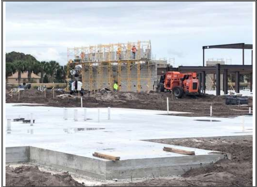
Photo 7 – View of newly poured concrete slab.
