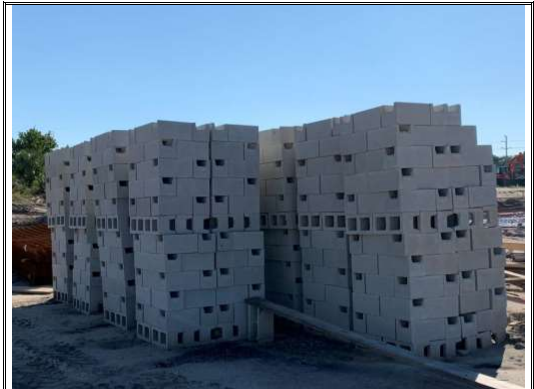
Photo 12 – CMU is on-site.
