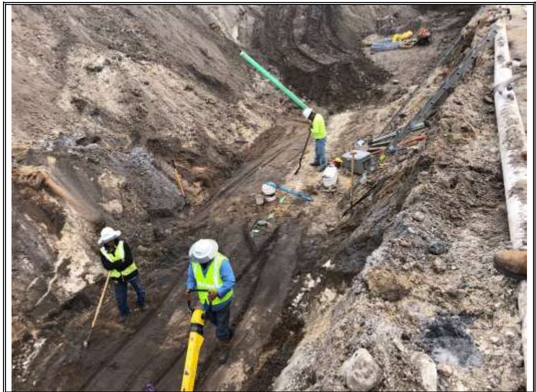
Photo 8 – View of ongoing sitework.
