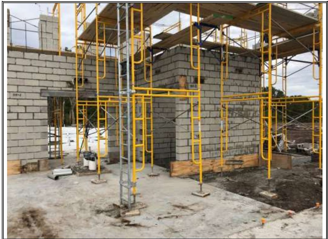
Photo 6 – CMU installation is ongoing at the main building.
