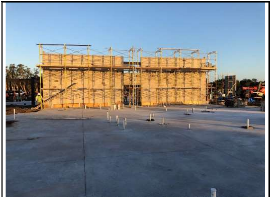
Photo 4 – View of scaffold erection and ongoing CMU installation.
