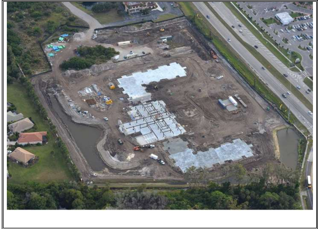
Photo 3 – Aerial view of the project. (Photograph provided by GC)
