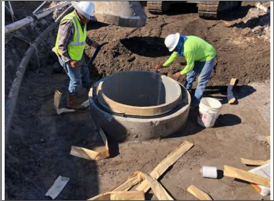
Photo 9 – Drainage installation is advancing.
