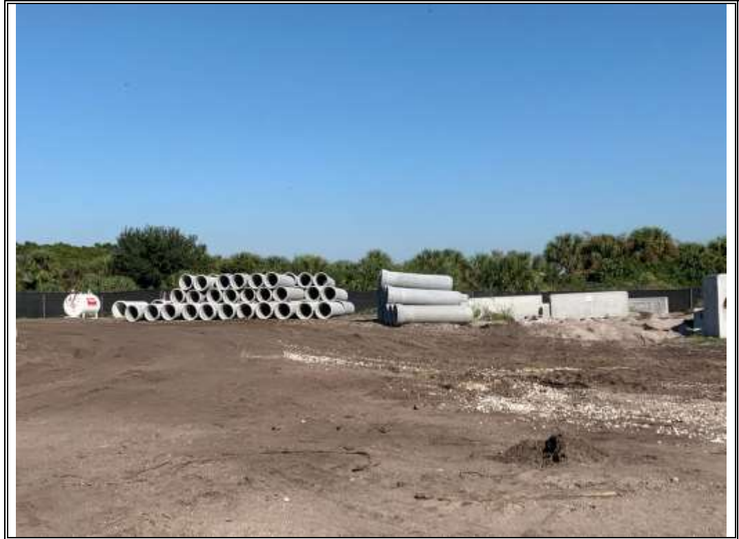
Photo 11 – Drainage piping is on-site.
