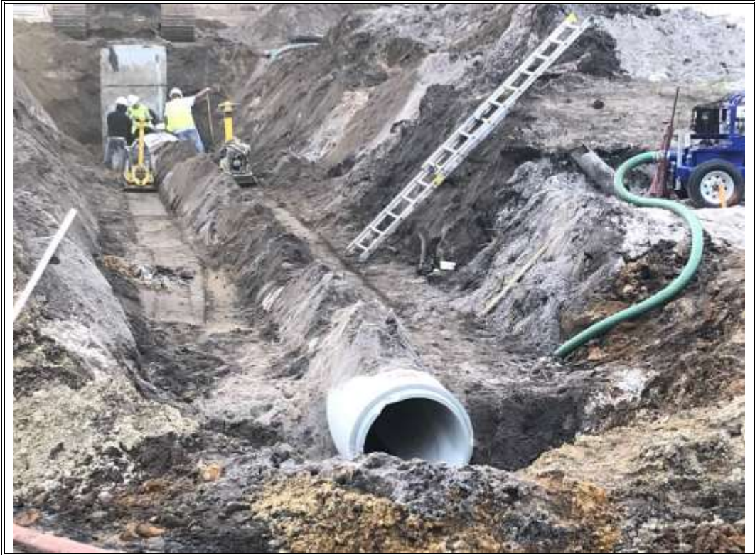
Photo 10 – Drainage installation is advancing.
