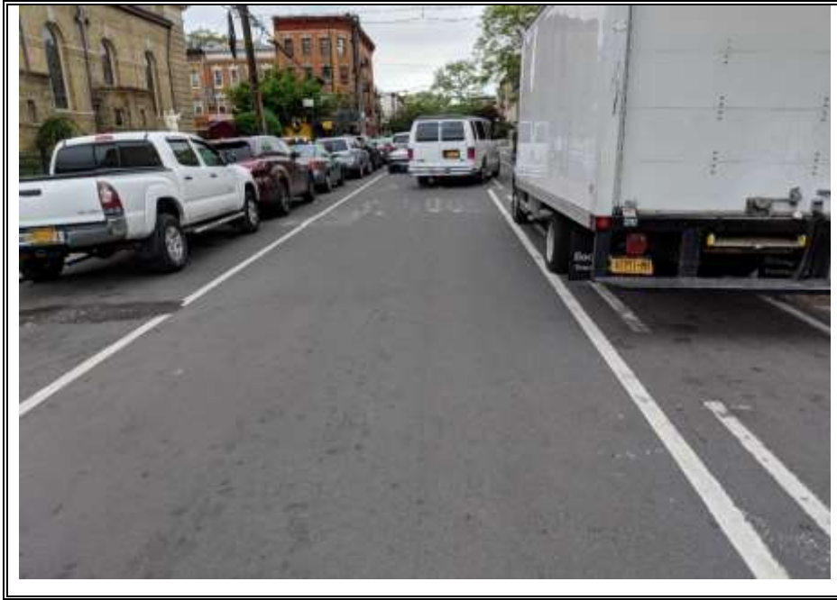
Photo 9 – The street is in good condition.
