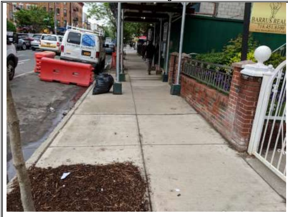
Photo 10 – The sidewalk and curbing are in good to fair condition.
