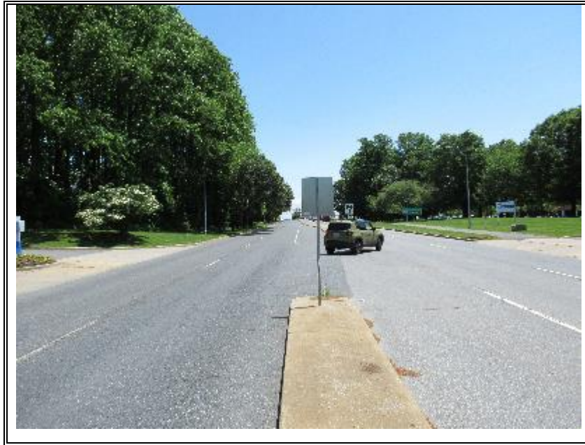
Photo 3 – East view of Commack Road in front of entrance.
